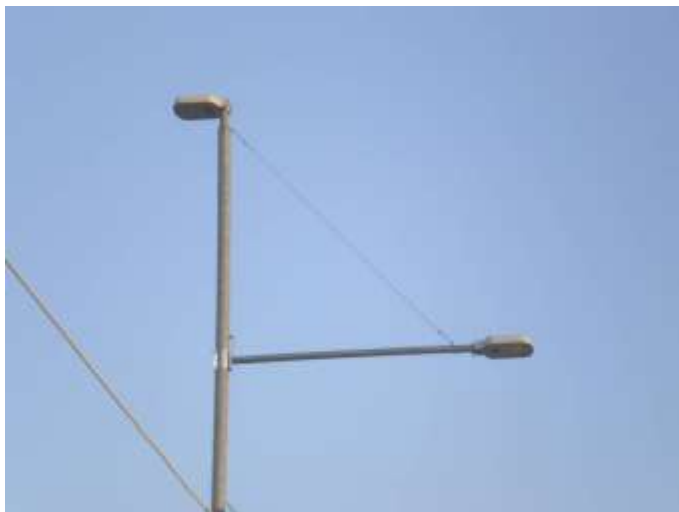
Slika 7. Philips ClearWay BGP303 LED49 3S/740 PSU I 4260 - 43W i Philips ClearWay BGP303 LED98-3S/740PSR II D9 76 - 81 W
