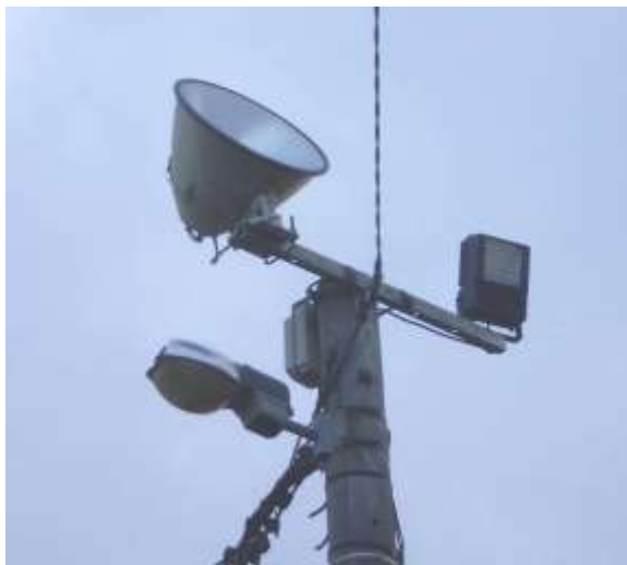
Slika 9. Gamalux LVC 06 150W NAV-E, reflektor LVR 507 250W HQI i LVR 09 150W HQI
